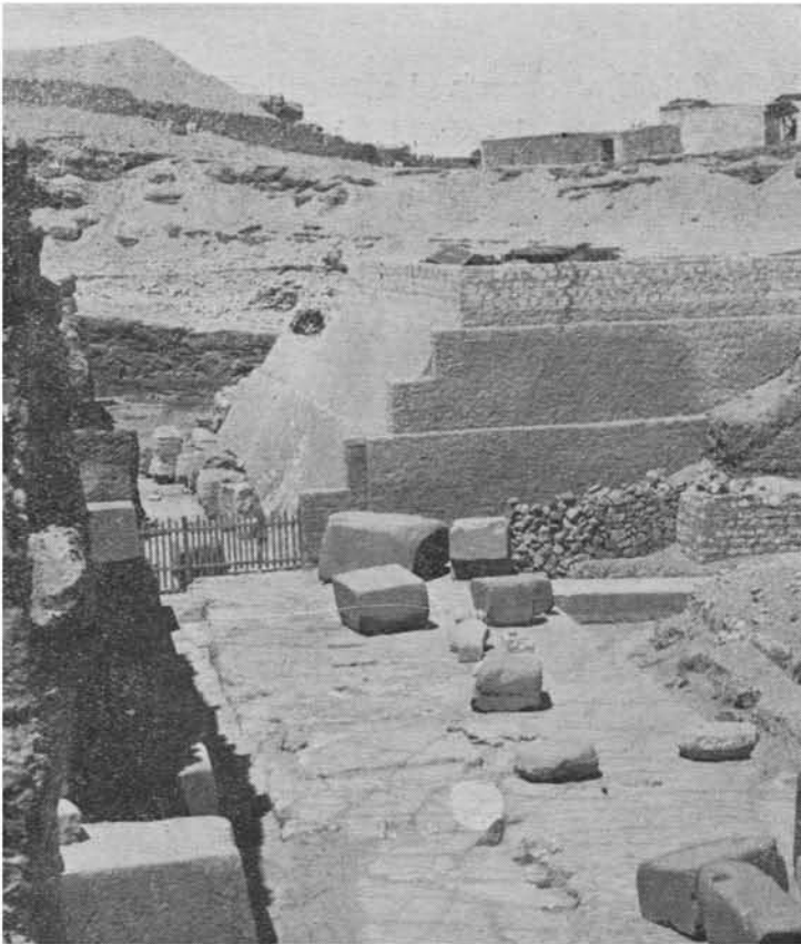
FIG. 10.—THE EASTERN PROTECTIVE WALL BUILT BY M. BARAIZE
