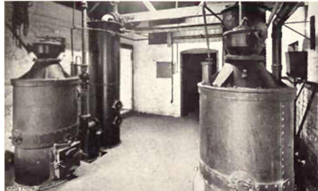
Photograph 4. Suction Gas Producers at Canwell. From Country House and Its Equipment, L. Weaver, Country Life 1912.
