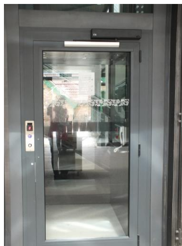
Lift to the Ticket Office
