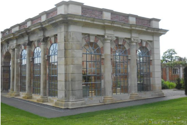
Orangery, showing wheelchair accessible route
