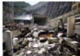
Destruction of hydro plant due to faulty M2M communications.
