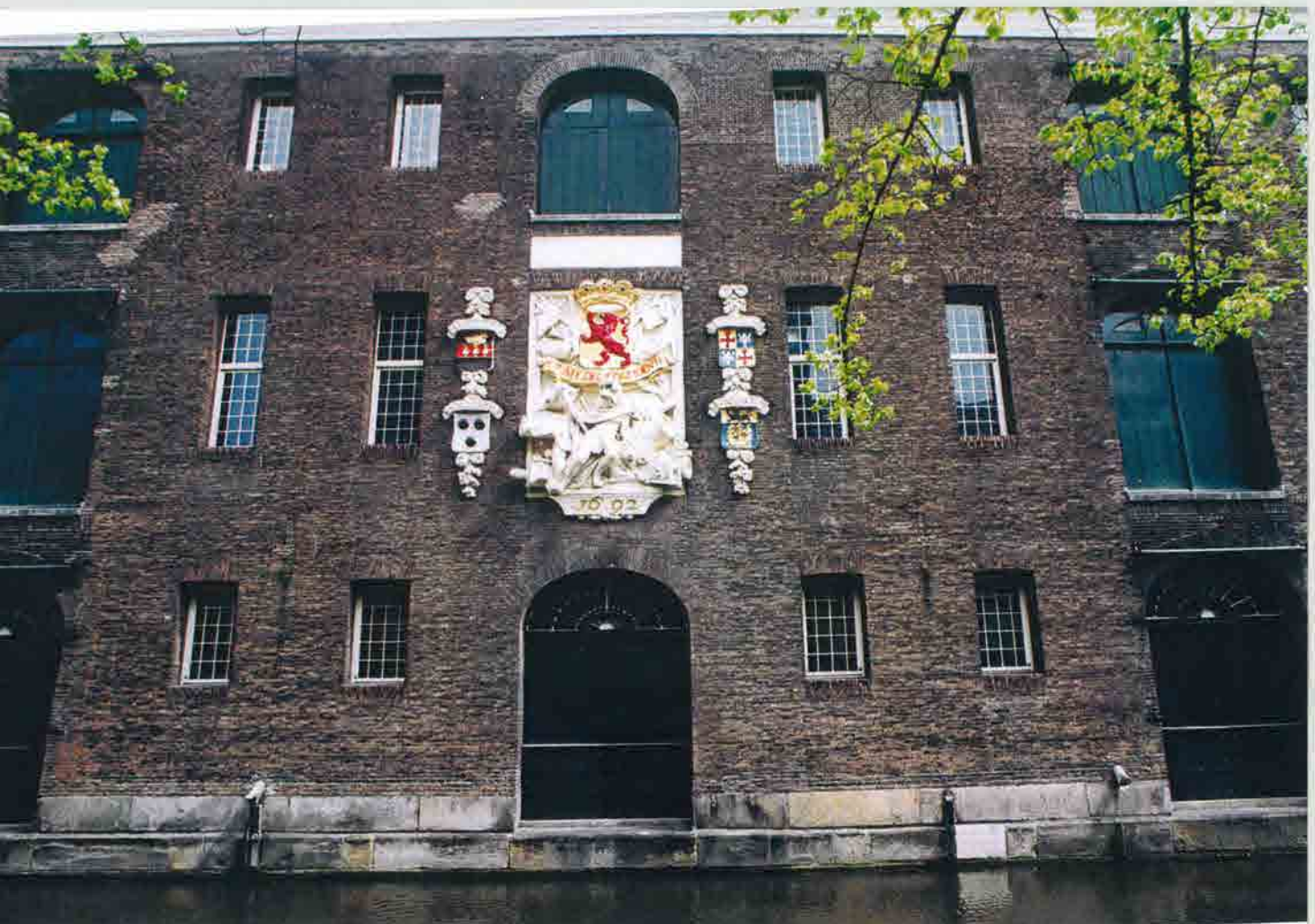
The original entrances to the old Armamentarium on the Oude Delft Canal.
