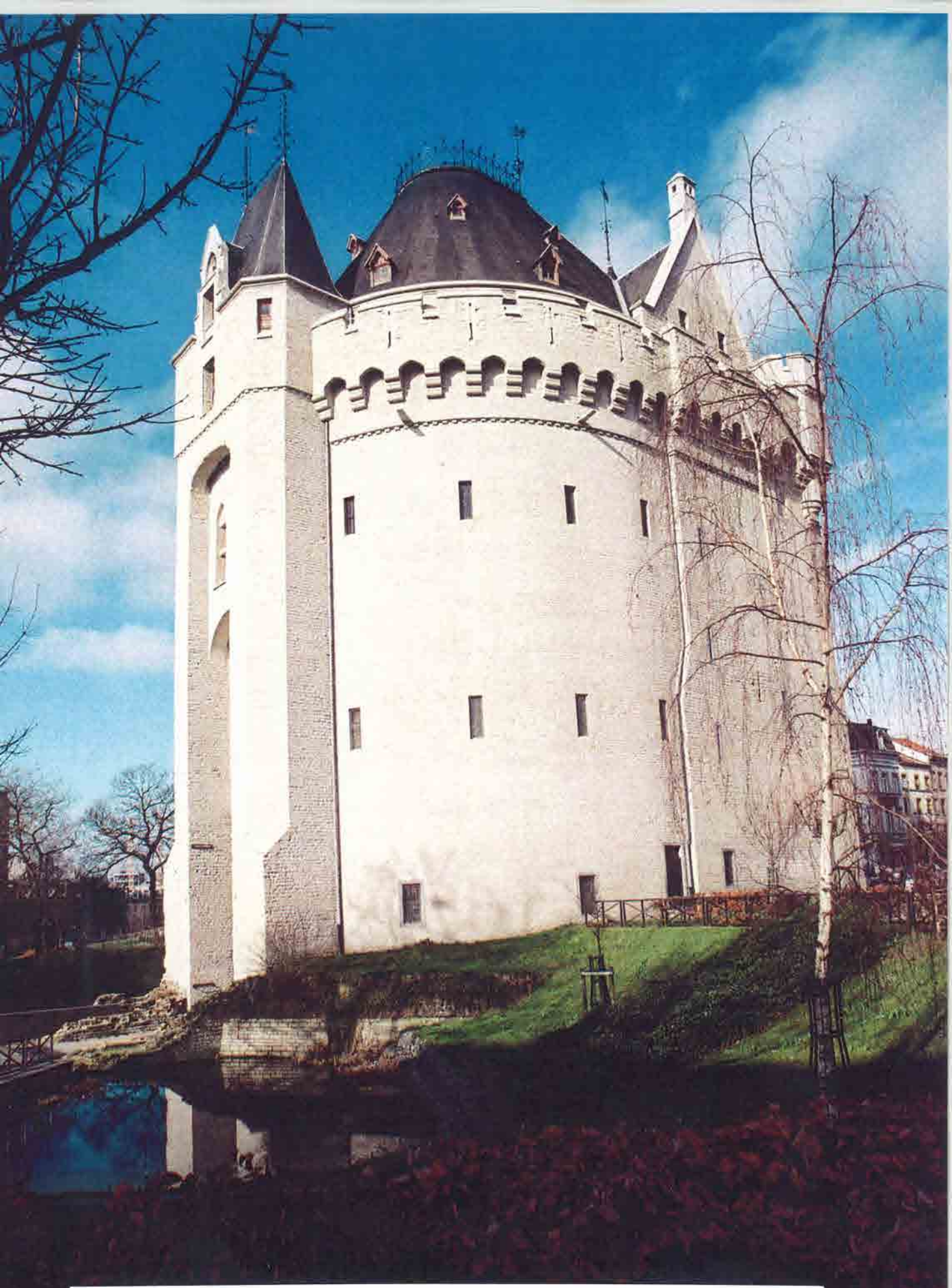
THE HAL GATE which formerly housed the Artillery Museum, now transferred to the Royal Army and Military History Museum. Note the small pond, all that remains of the original moat of the city walled fortifications.
