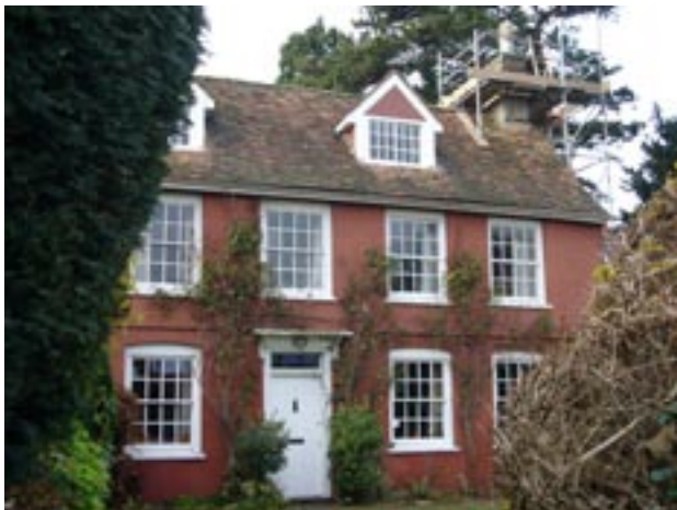
Red House, No 16 Church Street
