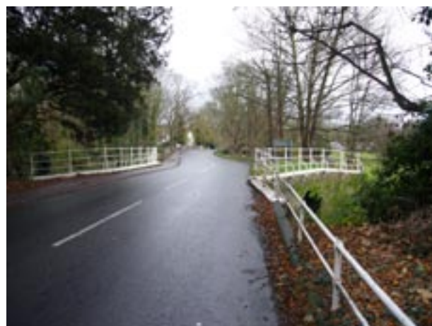
Bridges over the River Cam at the western edge of the conservation area
