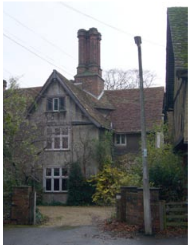
The Grange, Church Street
