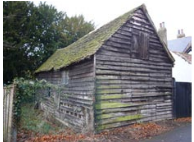
Apple loft and stables at rear of 33 Church Street
