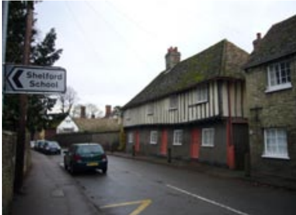
Nos 15 to 19 Church Street, the former parish guildhall
