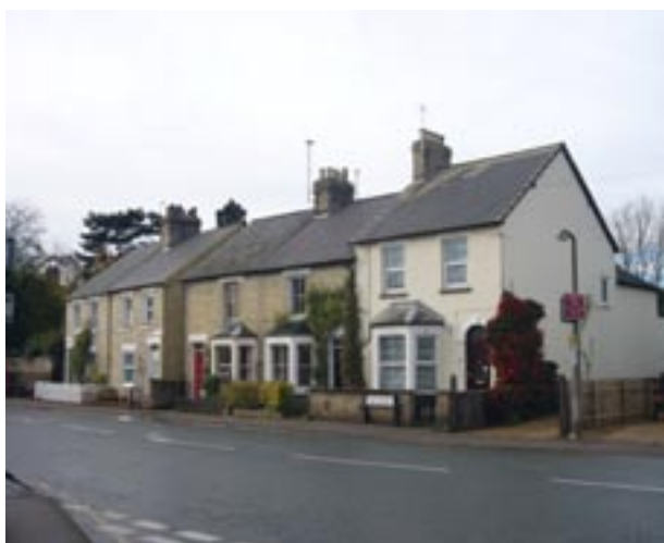
Nos 2 to 10 Church Street
