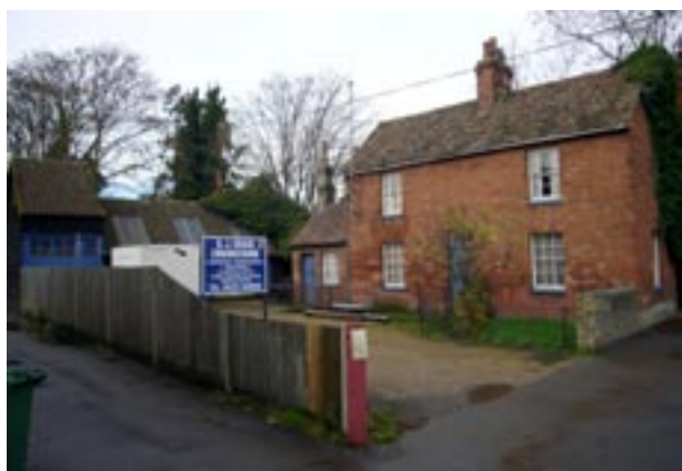
The smithy and house at No. 11 High Green
