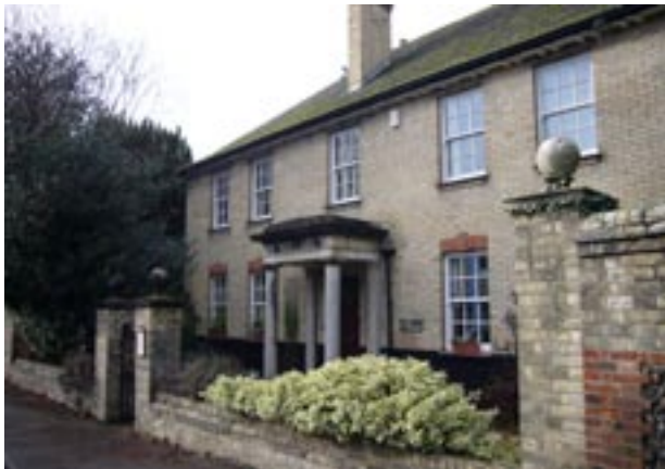
The Vicarage, No. 14 Church Street
