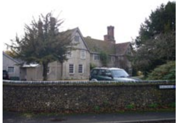
The Grange, Church Street
