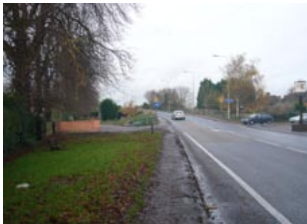
High Green: the approach to the railway bridge looking north, with vestiges of the former green in the form of wide verges to the left
