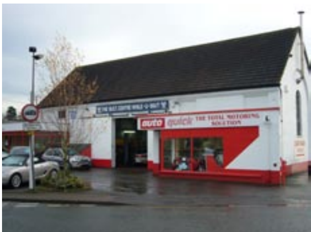
Junction of Church Street and Woollards Lane: former British School of 1845, converted to a garage in 1956
