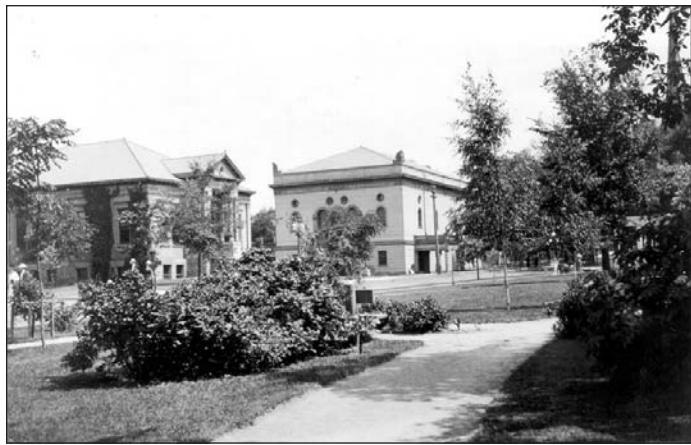
View of Carnegie-Lawther Library and T.B. Sheldon Auditorium, 1910's.
