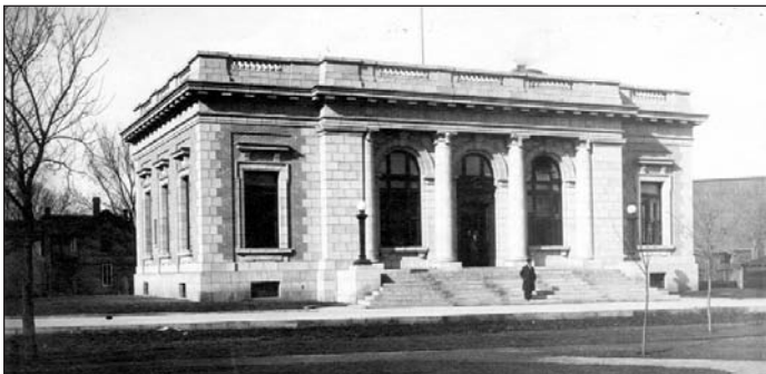
Red Wing Post Office, constructed 1906
