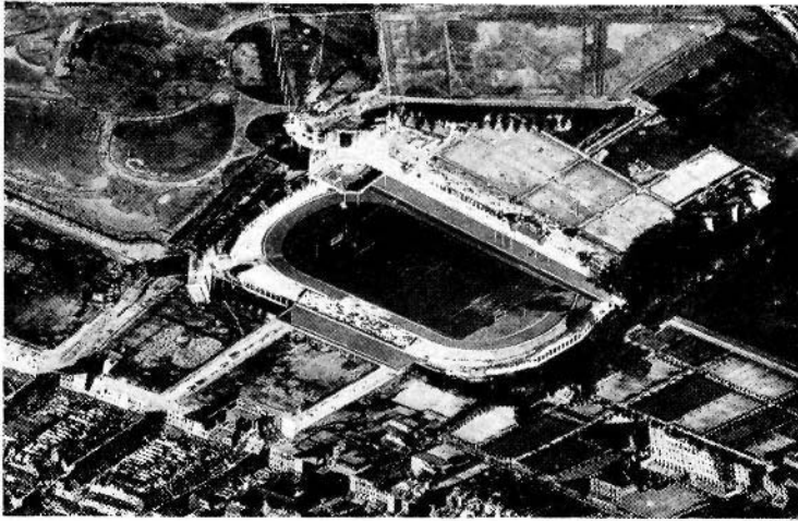
View of Olympic Stadium from Airplane
