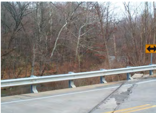
Existing guardrail and bridge condition
