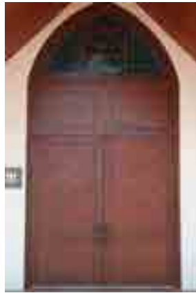
Timber door with stained glass window
