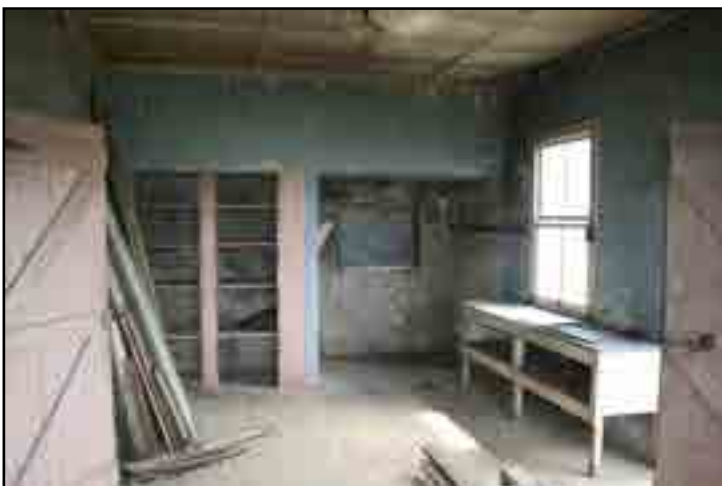
Kitchen has blue paint, sink, stove and shelving recesses
