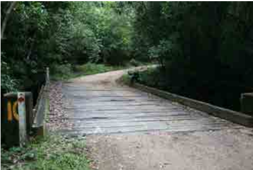
Kirrama Range Road: Bridge 10
