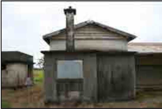
End of kitchen with stove and shelving recesses
