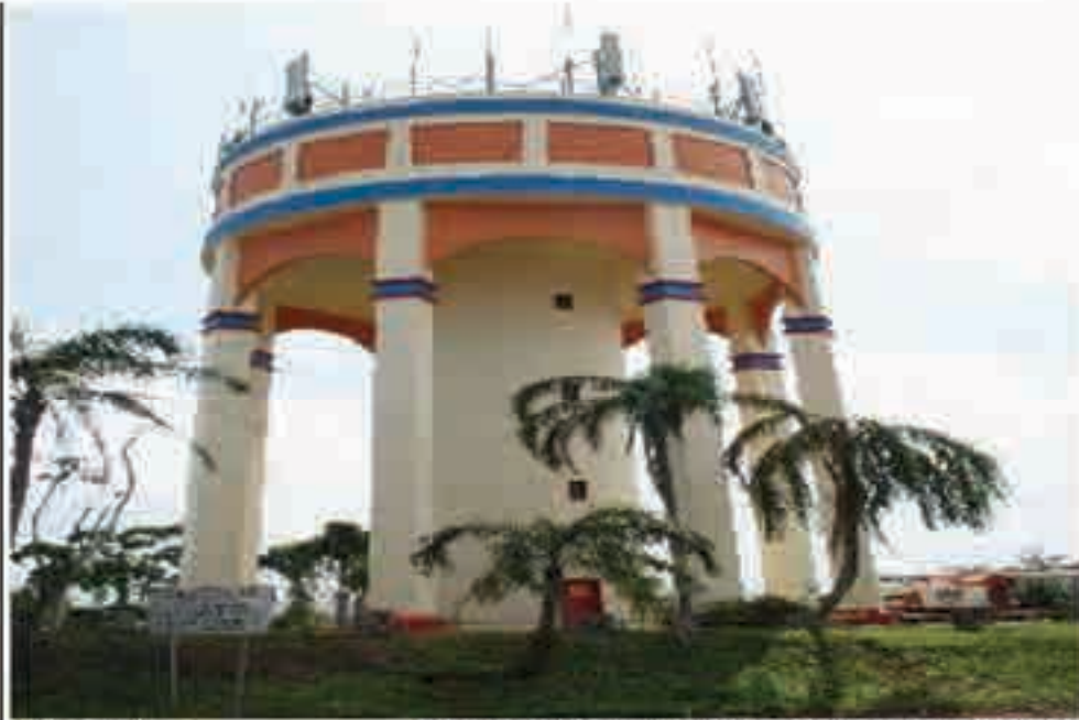
Description View of Innisfail Water Tower from Mourilyan Road (2011). Media Author Cathy Browning Media Date 30/03/2011 Copyright DERM
