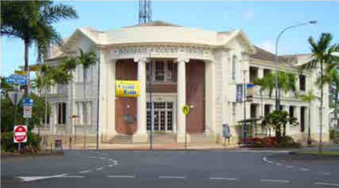
Innisfail Court House
