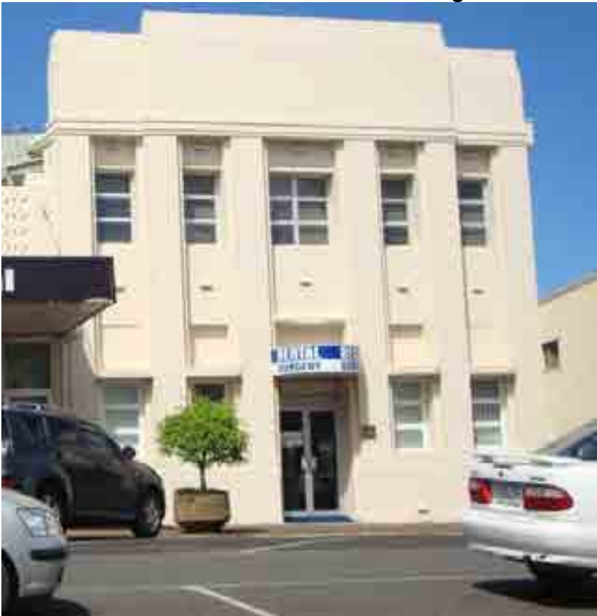
Former Queensland National Bank Building
