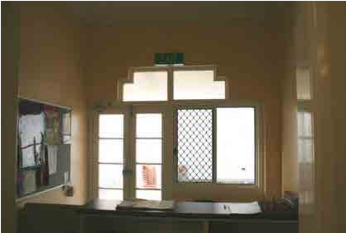
Window at front verandah area
