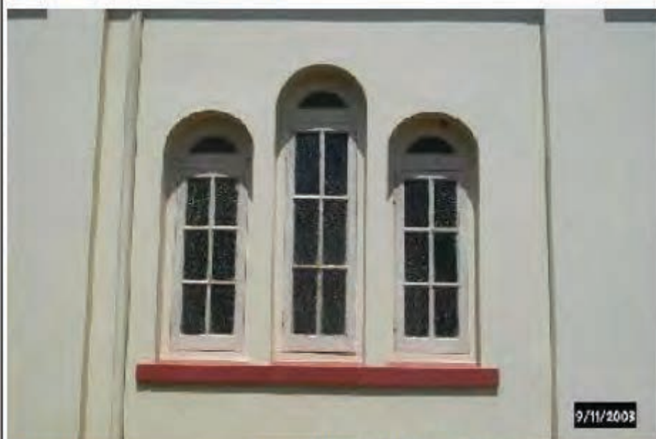
Description Former St Saviour's Anglican Church
