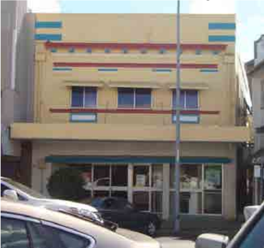
Former National Bank of Australasia Building
