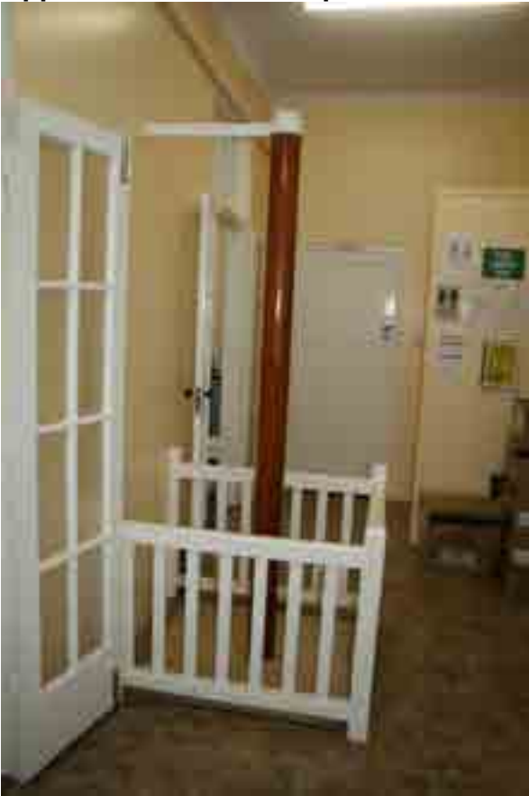
Upper end of fireman's pole
