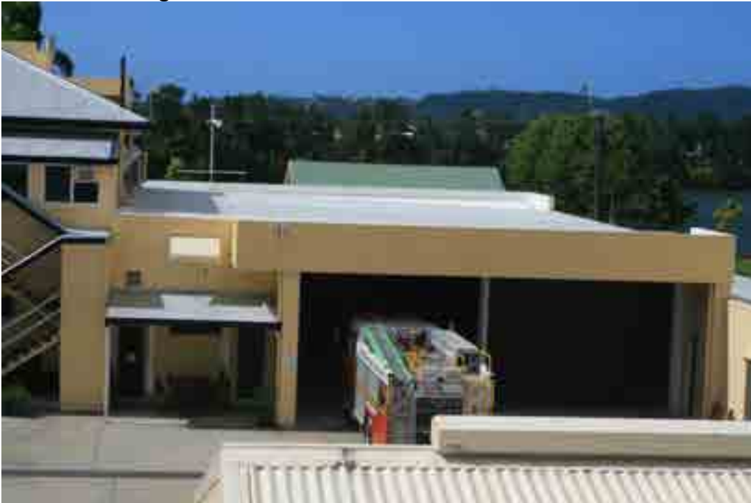
Rear of building - new section
