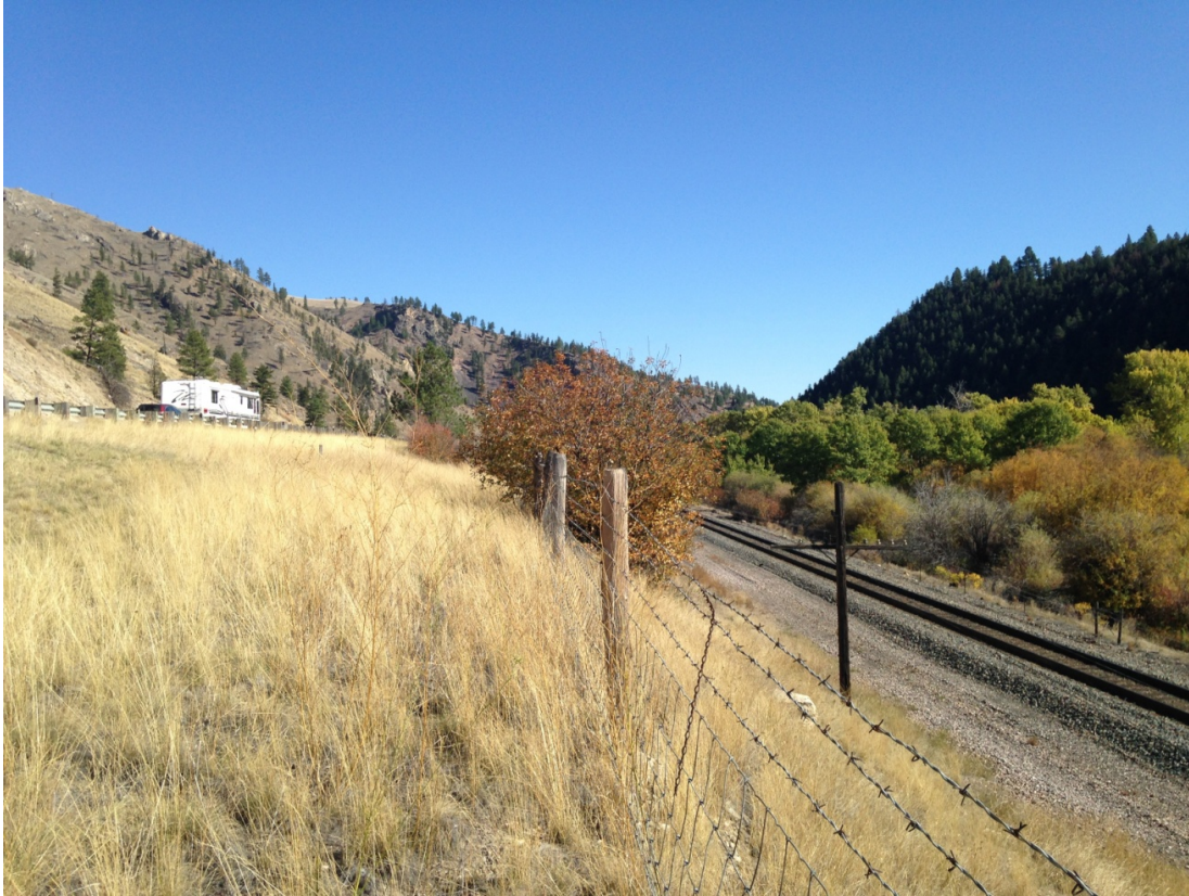
Figure 25. Poor opportunities for mitigation at site 4a. Photo taken Oct. 10, 2014 by M. McClure at milepost 136.
