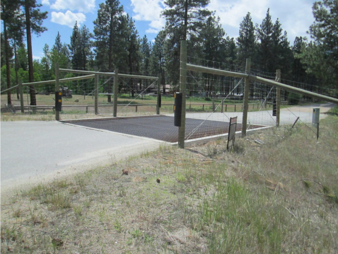
Figure 15. Wing fencing and cattle guards with adjacent perpendicular fencing are designed to keep animals from entering the roadway between crossing structures. Photo taken June 2, 2014 by M. McClure at US-93 and St. Mary's Road, Stevensville, MT.
