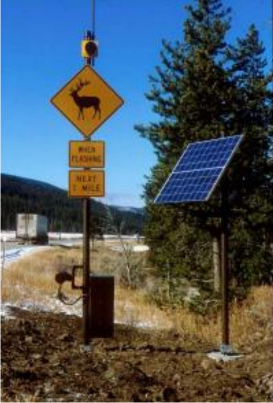
Figure 17. An animal detection system (ADS), which alerts drivers to the presence of wildlife on or approaching the road (Photo courtesy of Marcel Huijser).
