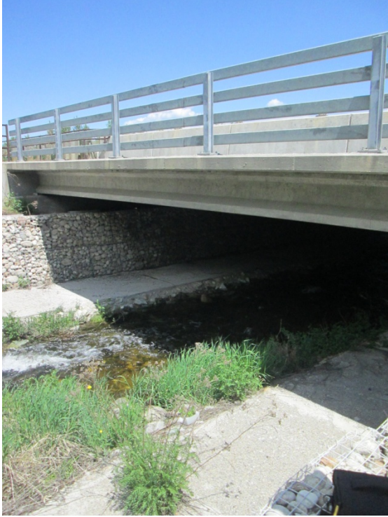
Figure 20. Example of stream crossing that is also designed as a wildlife underpass. Photo taken June 2, 2014 by M. McClure on US-93 between Hamilton and Stevensville, MT.
