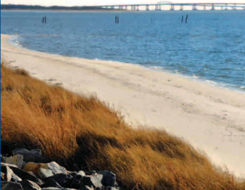
Chesapeake Bay Bridge-Tunnel viewed from Virginia
