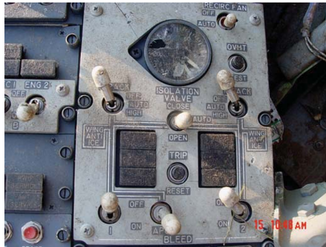
Photo – Air Conditioning Panel
