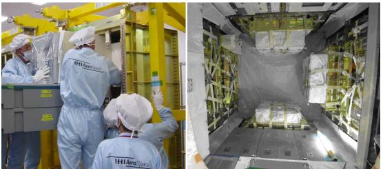
Figure 4.1-3 CTBs being installed in an HRR Right: HRRs being installed in the PLC (HTV2)\* \*This photo was taken during the cargo loading process. More CTBs are to be added later at the front of the HRR.
