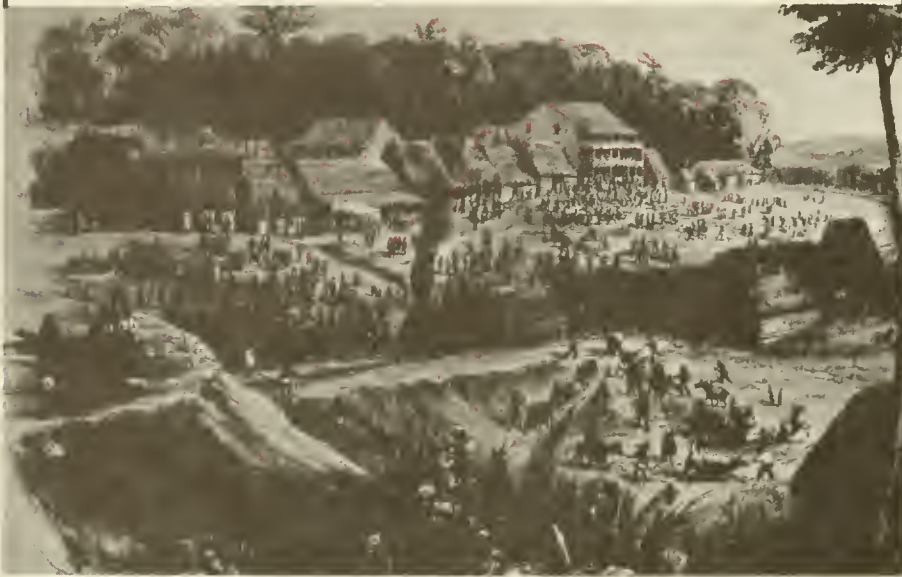
All was chaos at Culebra where the railroad ended in 1854. This painting by Otis M. D. Surgeon shows work proceeding on the railroad, at left, while in the foreground California-bound travelers round up burros and mules to continue their overland trek. Crowds of stranded Forty-niners fill the balconies of the American Hotel at the far right.
