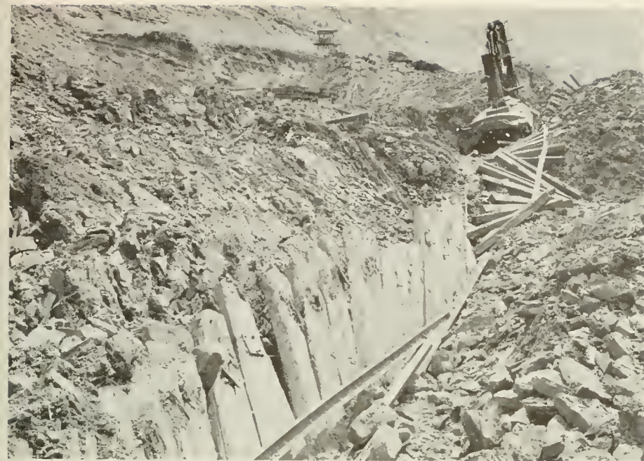
A sample of what happened to the early Canal diggers from time to time. A break in the east bank at Culebra in 1913 poured material into the bottom of the Cut tearing up railroad tracks and burying a steam shovel. Some buildings had to be moved from the side of the Cut.
