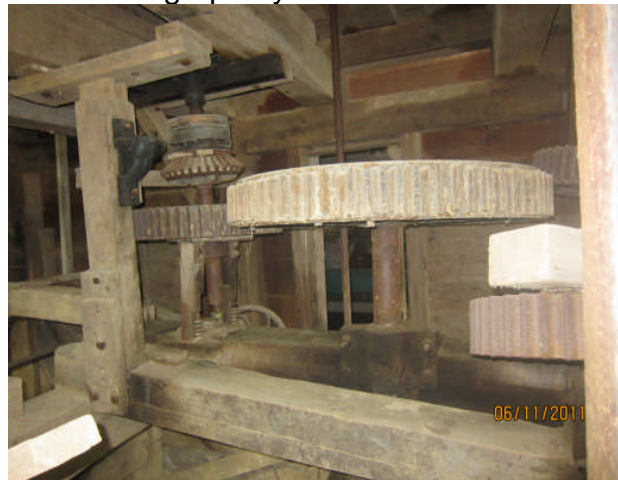
Bair’s Mill Turbine June 13, 2011 Photograph by James C. Strickler
