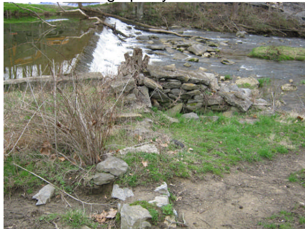
Remaining Foundation of the Original Strickler's Mill at Bair's Mill April 10, 2011 Photograph by the Author
