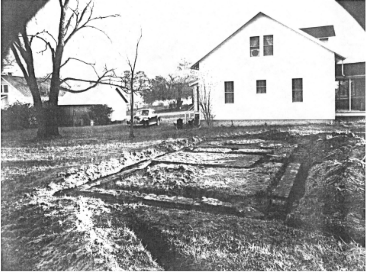
Figure 10. Foundation of laundry/kitchen.
