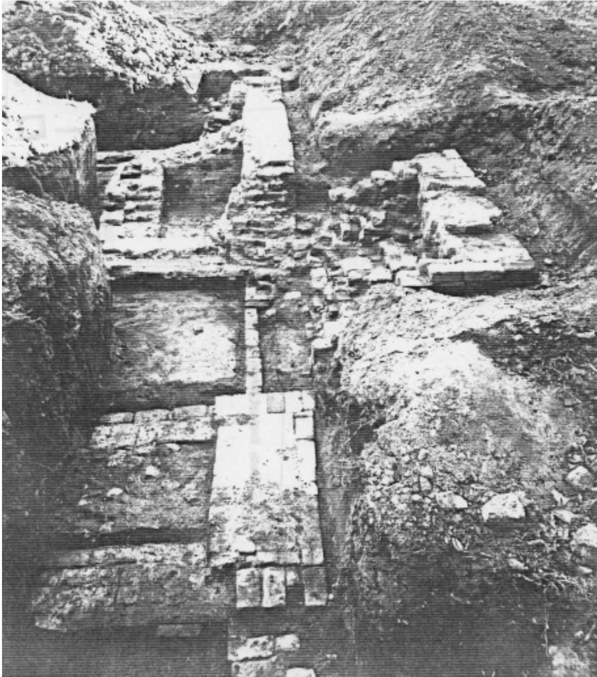
Figure 7. West foundation wall of main house.
