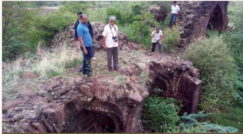
Deputy Commissioner, D. Randeep looking at the ancient water system during his recent visit.
