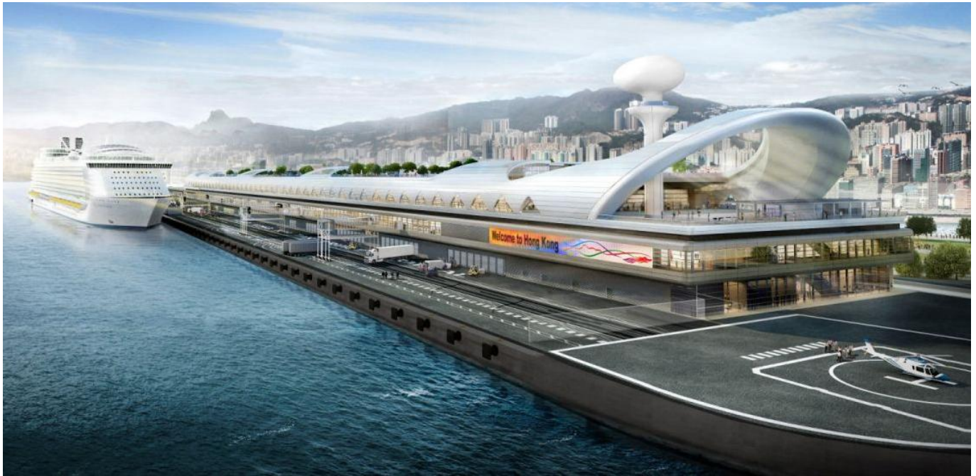
▲ The new Cruise Terminal Building in Hong Kong is able to accommodate two 'mega' cruise ships. Its features include large column-free spans and the largest roof-top garden in Hong Kong, with incredible views of Hong Kong Island and the Kowloon Peninsula.
