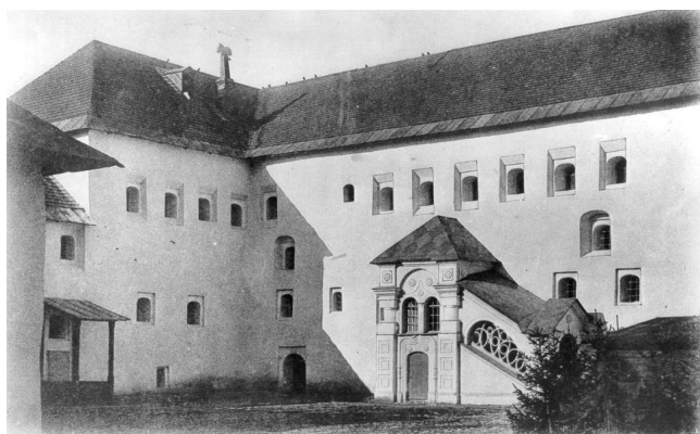
Pogankin Chambers. View from the courtyard. Photo early 20 th century.
