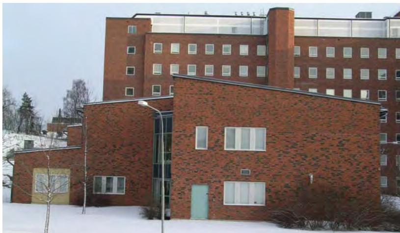
Uppbrutna former. SBA D20040129-021
