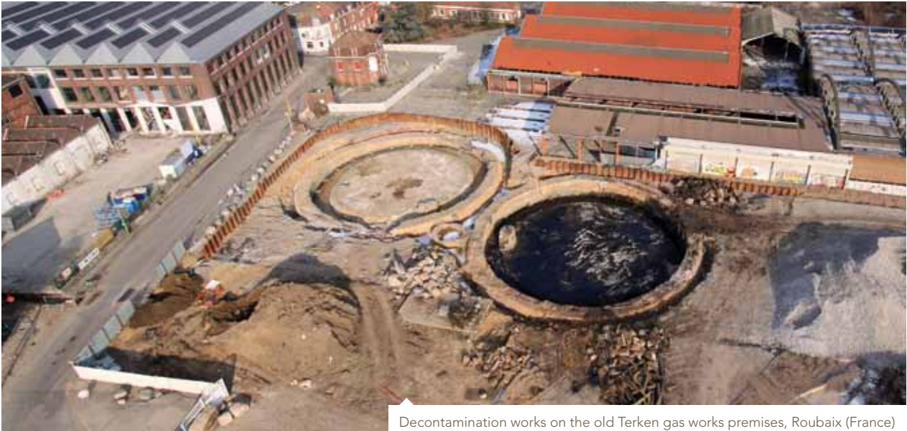
Decontamination works on the old Terken gas works premises, Roubaix (France)
