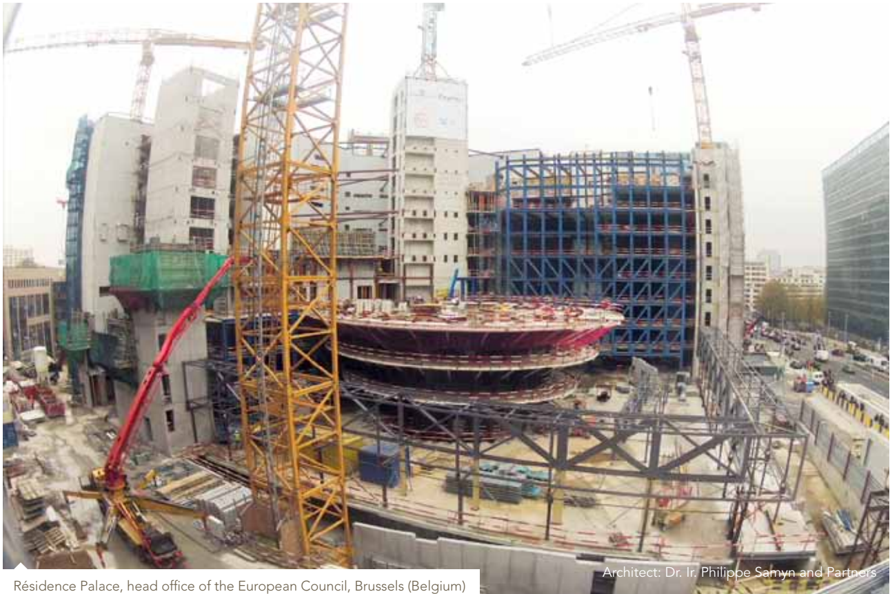
Résidence Palace, head office of the European Council, Brussels (Belgium)
