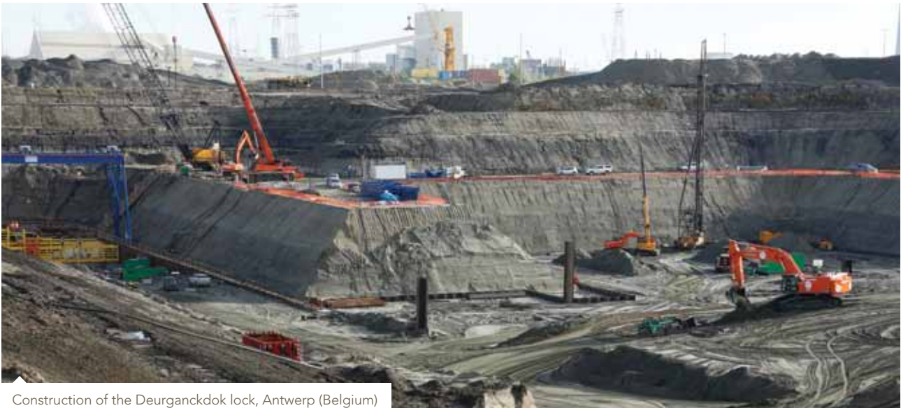
Construction of the Deurganckdok lock, Antwerp (Belgium)
