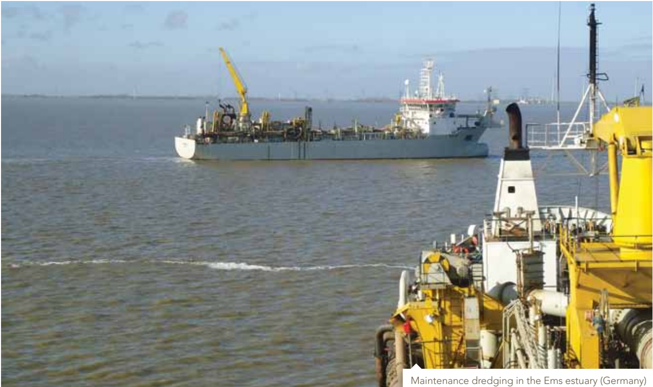
Maintenance dredging in the Ems estuary (Germany)
