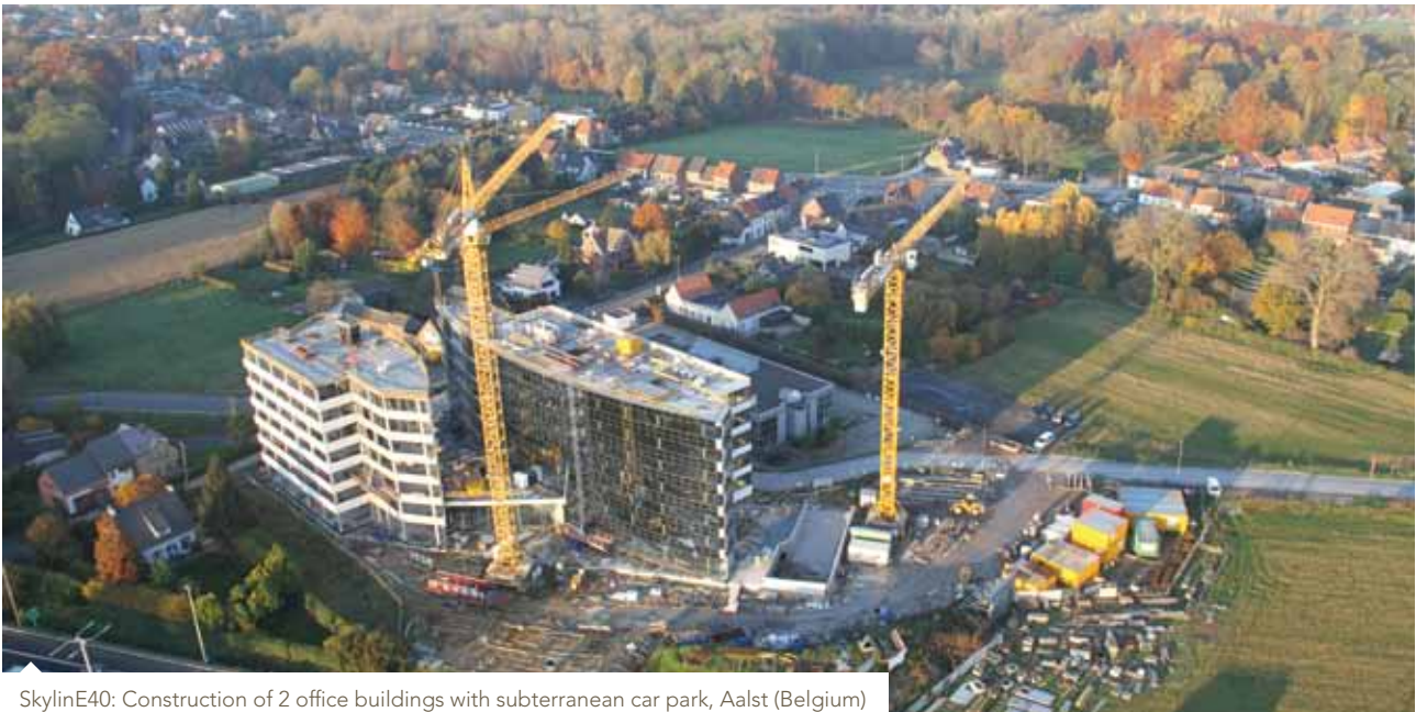
SkylinE40: Construction of 2 office buildings with subterranean car park, Aalst (Belgium)
