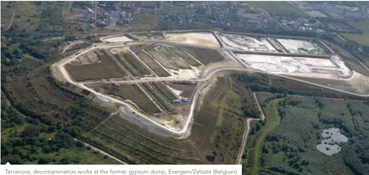
Terranova, decontamination works at the former gypsum dump, Evergem/Zelzate (Belgium)
