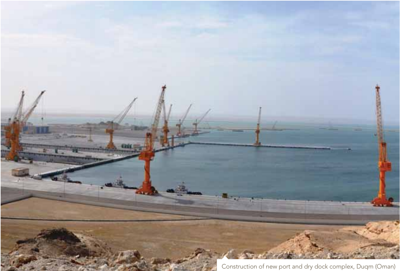
Construction of new port and dry dock complex, Duqm (Oman)
