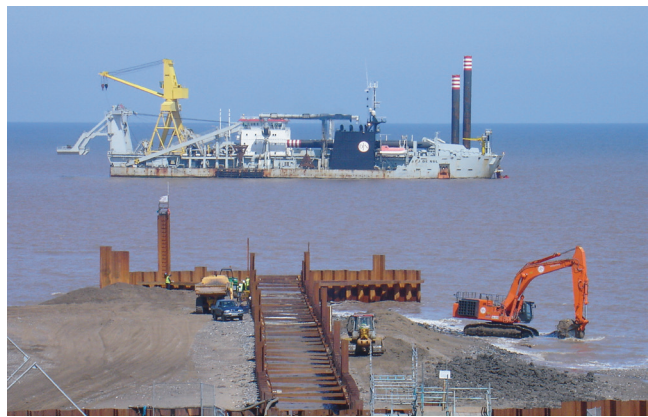
Figure 6. The cutter dredger J.F.J. De Nul in front of a typical cofferdam construction.
