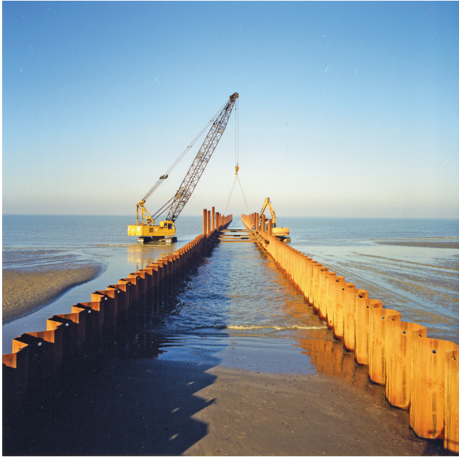
Figure 5. A typical cofferdam construction.
