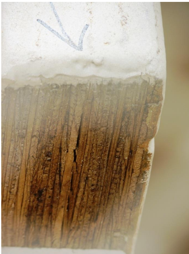
Fig. 17 Sprayed-on Polyurethane-2K-coating with beige top coating
