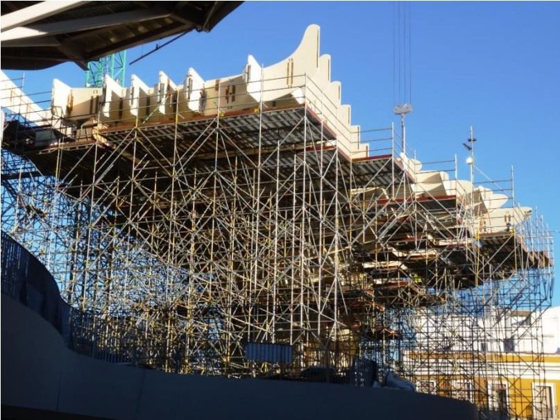
Fig. 21 Construction of the scaffolding for the cap assembly
