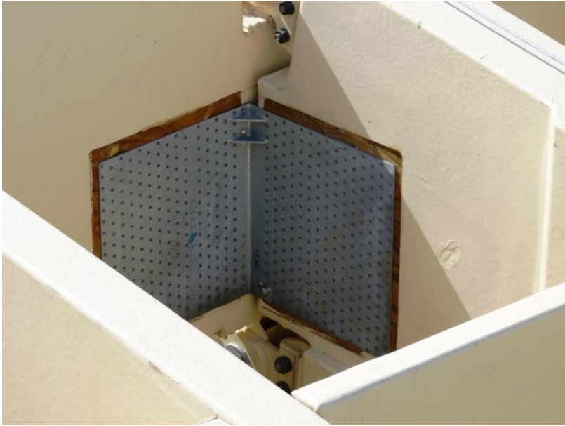
Fig. 13 Angled connector plate to transfer shear forces
