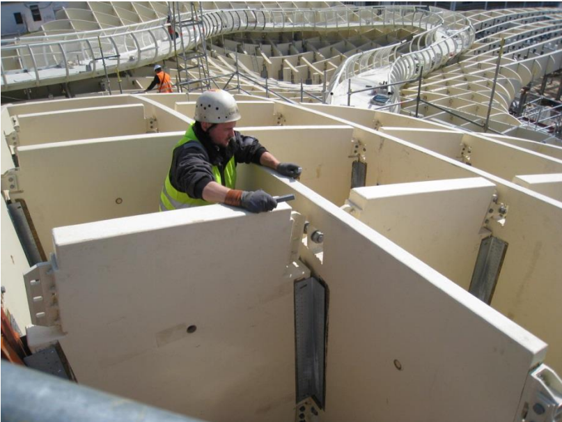
Fig. 22 Connecting the timber beams
