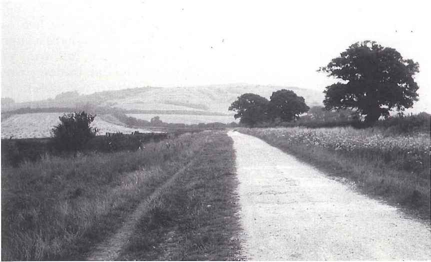
3 The Old Bath Road, seen here as a track over Roundway Down. The foreground shows the narrow turnpike road flanked by drainage ditches, with verges cleared of vegetation to deny cover to highwaymen.
