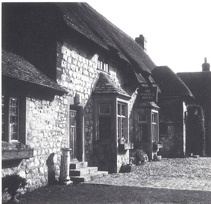
9 The Waggon and Horses , Beckhampton, typical of the older-style inns on the road.
