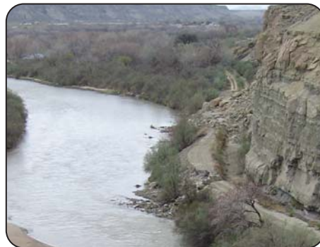
Passed in 2009, Public Law 111-11 authorized $7 million to repair unstable rock formations near Farmington, New Mexico. Heavy equipment in the San Juan River needed to repair the slides threatens critical habitat.
