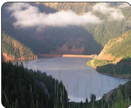
Coordinated releases from Ruedi and other Colorado reservoirs enhance spring peak flows in the Colorado River for the endangered fishes. Combined releases in 2009 of 42,783 acre-feet were the highest since the Coordinated Reservoir Operations Program began in 1995.
