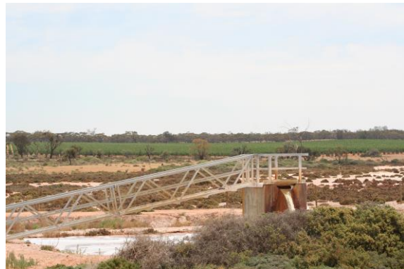
Mourquong disposal basin at Buronga, NSW Photo: Alison Reid, MDBA
