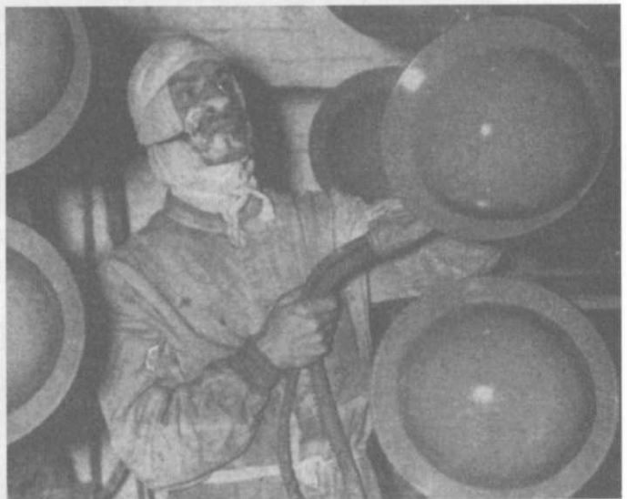
Above left, a helmet has just been stamped out of a blank and the operator holds in his hand the surplus metal. When once the helmet has taken its final shape it is painted inside and outside before the linings are put in. Right, a man is spraying on the paint. He wears a mask over his mouth and nose to guard against inhaling particles of paint, while his hair is protected from the spray by bandages. After being painted, the helmets are passed on a conveyor through drying furnaces.
