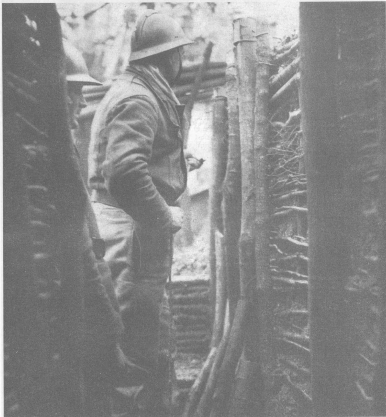
This scene is in a forward listening post of the French defences in front of the Maginot Line. Very notable is the strong brushwood and timber revetting of the trench. Here there is no chance of the parapet collapsing, as it sometimes did in the hastily dug trenches during the last war. The officer in the centre of the photograph is on a round of inspection. In page 426 is a diagram that shows the position of such a listening post in regard to the main defences of the Maginot Line itself.
