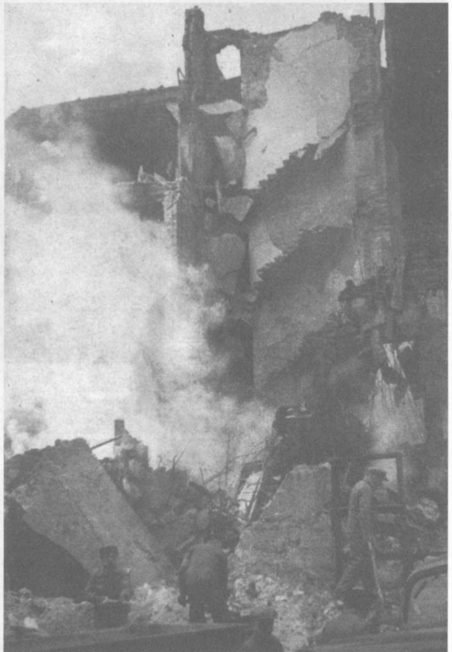
Here is the real thing—a scene in Helsinki during one of the Red Air Force's raids in the opening days of the war in Finland. An high-explosive bomb has been dropped on a four-storey house. Three of the walls have collapsed, and on that which still stands are the shattered remains of a staircase. Men are at work searching the debris.
