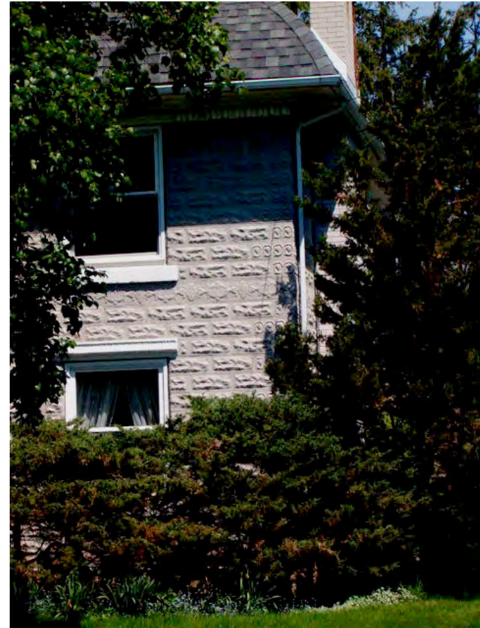
A detail of the ornamental blocks from the North American Cement Block and Tile Company, used here on George Baker's own house, across the road from his factory.
