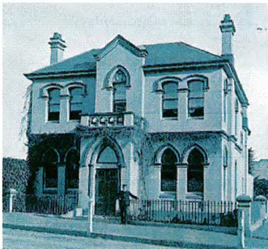
Figure 5 The 1885 C B C Bank building, now occupied by the National Australia Bank.
