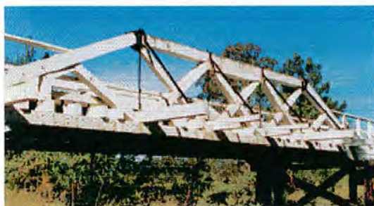
(a) Old PWD truss
