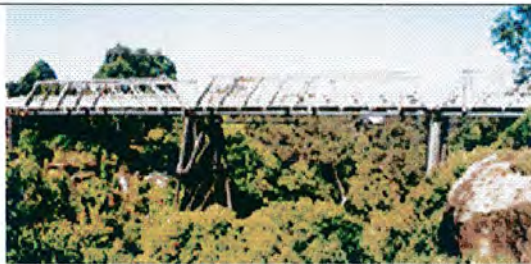
1897 Victoria Bridge over Stonequarry Creek, Picton.
