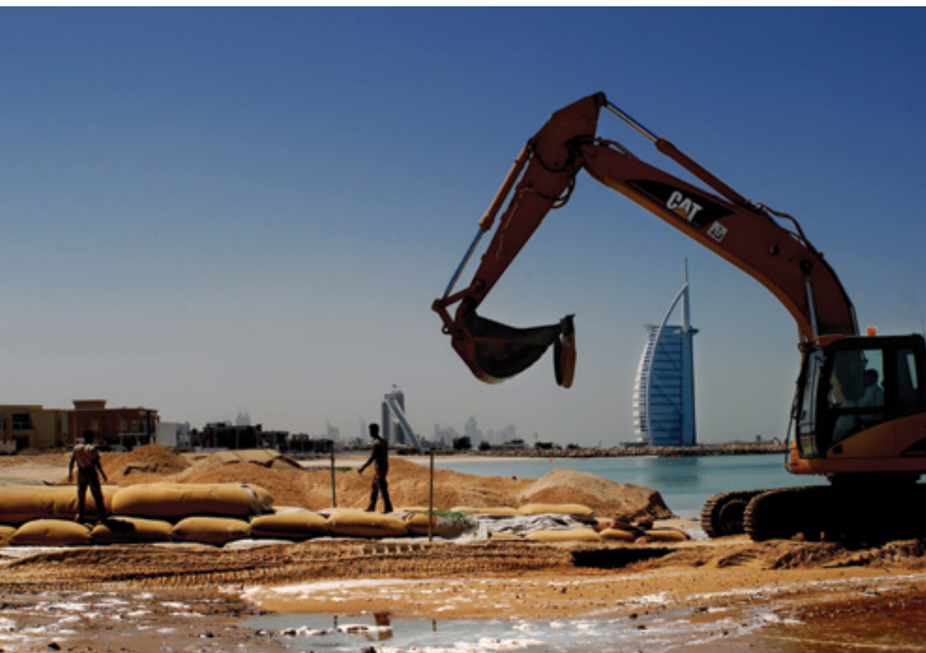
United Arab Emirates (UAE), Dubai. Migrant labourers working on extending the Dubai beach, close to the Burj Al Arab Hotel (right). The employers keep their employees' passports when they arrive and pay their workers around US$167 a month.
