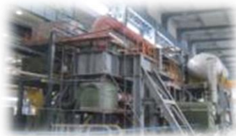
RCP test loop
