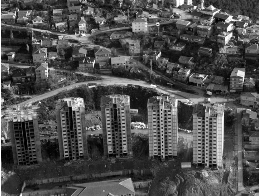
Figure 4.3 The first phase of the project is almost complete. November 2008 (photo credit: Nazim Akkoyunlu)
