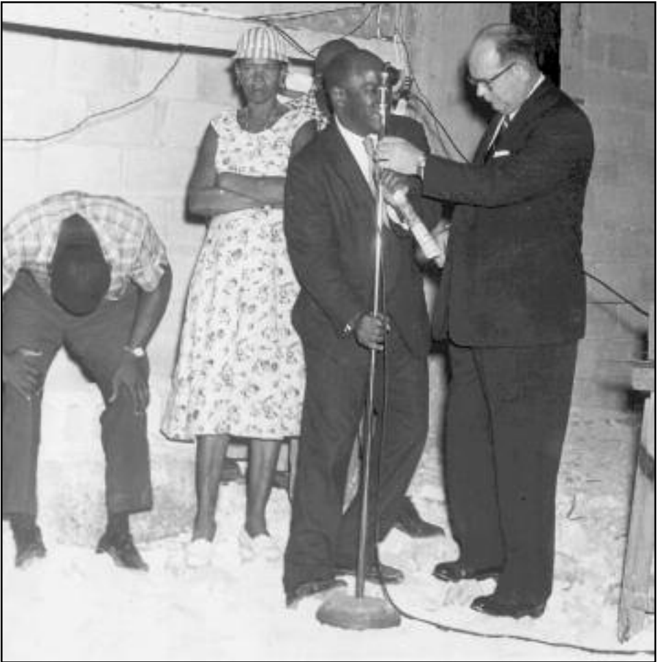
The author assists Ed Sullivan, President of New York's Building Services Union (AFL-CIO), as he prepares to speak in the gravel and debris found during the early stages of construction of the House of Labour. Marion Stuart stands in the background.
