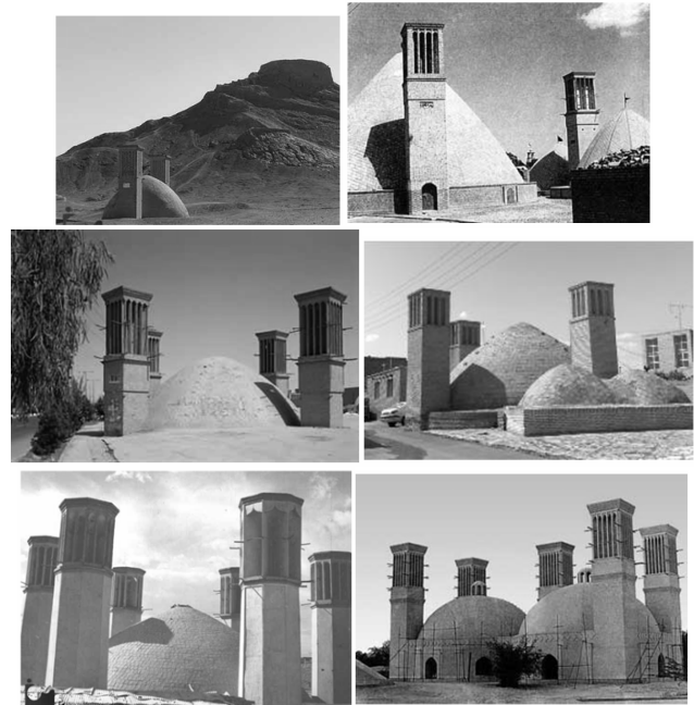
Fig.3. (right top) a one badgir towers, Naeen, (left top) two badgir towers, Kish, (right middle) three badgir towers, Isfahan, (left middle) four badgir towers, Yazd, (right below) five badgir towers, Kish, (left below) six badgir towers, Yazd, Iran, Ab Anbar.
