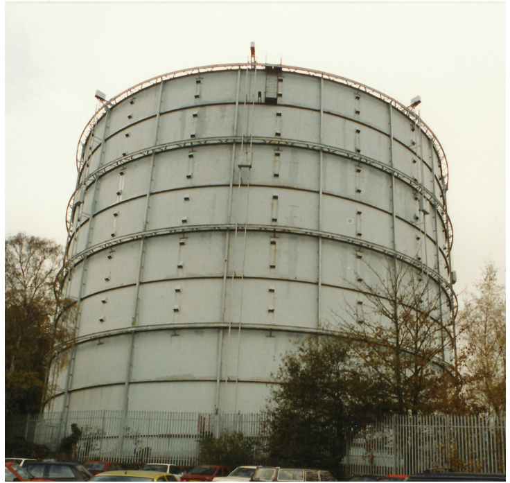
Low-pressure storage gasholder at Oxted.
