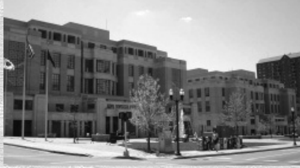
New Fayette Co. Courthouse
