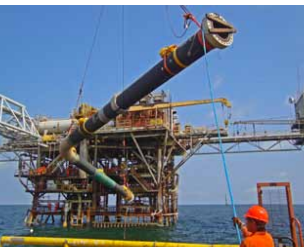
The installation of a spool piece, part of the SMIT Subsea Africa project in Nigeria.
