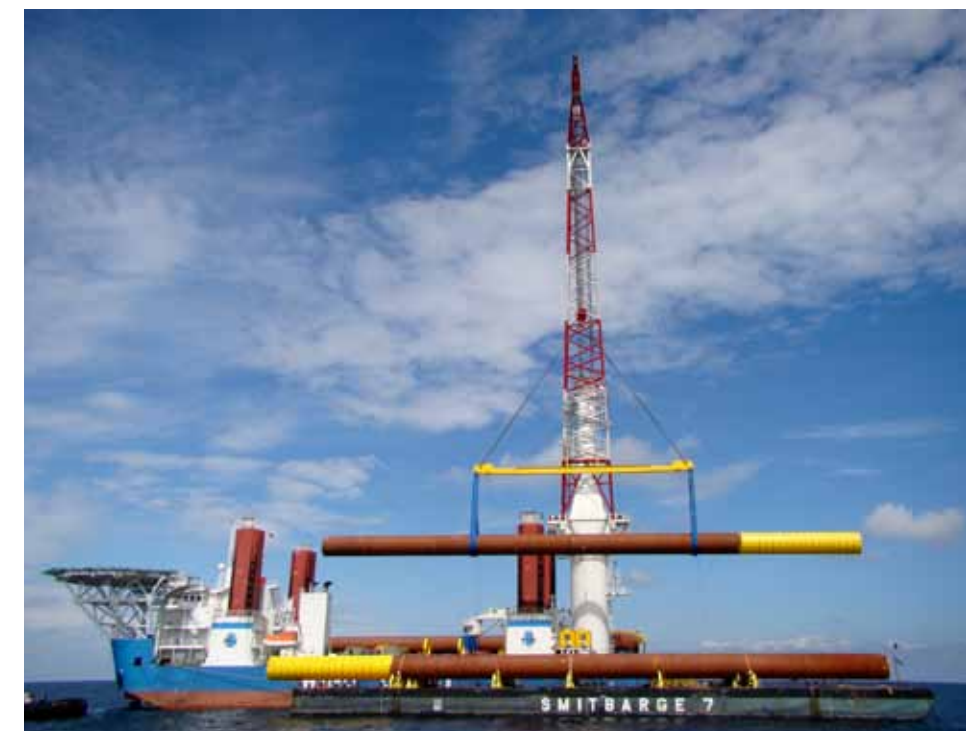
'Smitbarge 7' discharged by installation vessel 'Windlift 1' during the construction of Bard 1.
