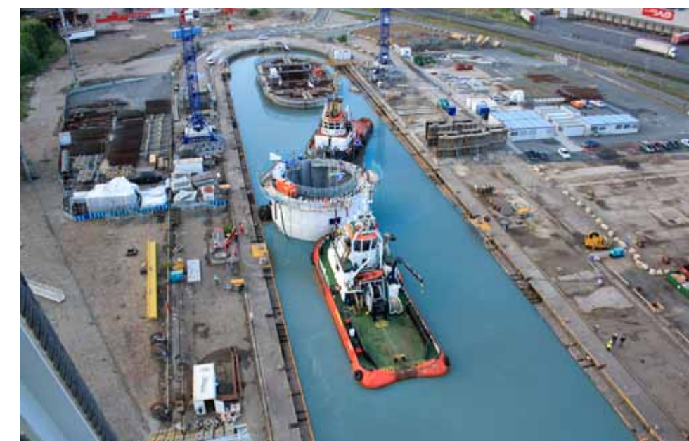
The 'Union Diamond' and 'Red Wolf' towing one of the caissons out of the dry-dock.
