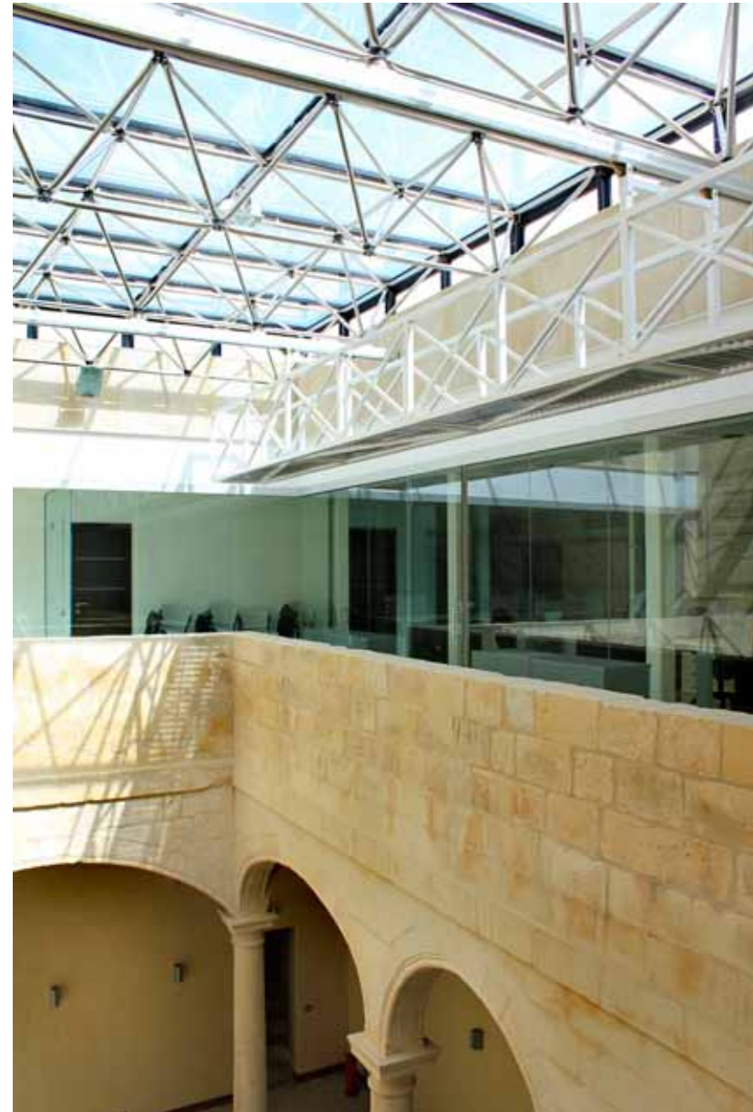
Lightweight space frame structure which shelters the courtyard
