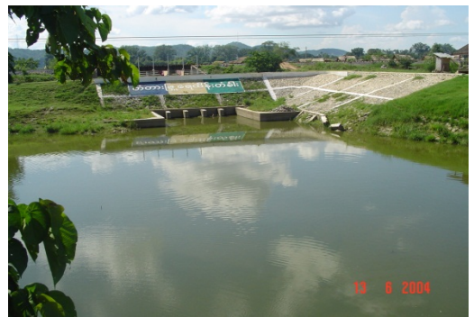
Fig 9. Tadarphyu sluice gate
