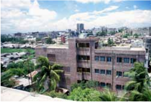
Deep Shikha Primary School, 1990 - 1998, © Aga Khan Trust for Culture - Aga Khan Award for Architecture / photography A.S. Kashef
