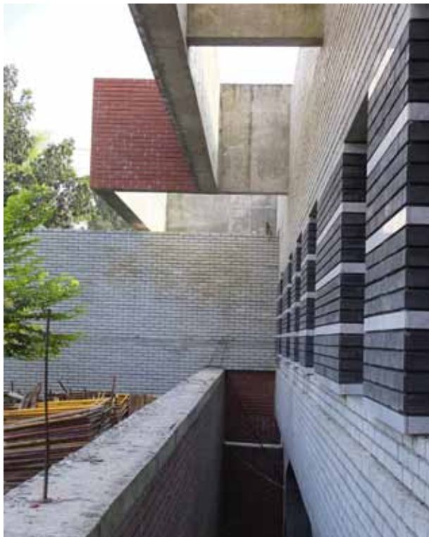
Franco-German embassy, Dhaka, detail during the construction, 2015, © AL
