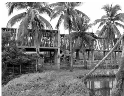
Olive Grove Children Home, Chokoria, view of the construction, ©Salauddin Ahmed
