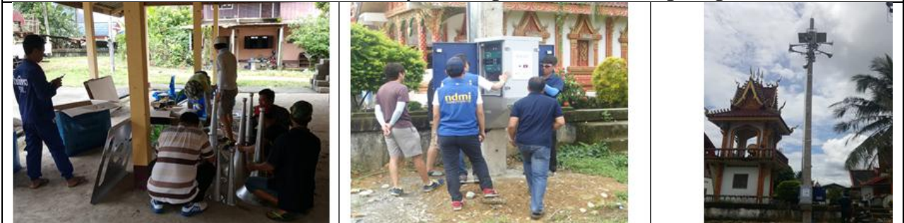
Automatic Flash Flood Early Warning Post at Ban Hua Yea
