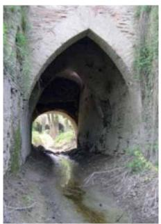
Fig.3 - On the left, south view of the Tower of Waters; the great ogival vault on the Galasso canal, which constitutes the foundation of the tower
