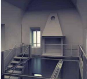
Fig.7 - On the left, the designed great cistern, repositioned at the extrados of the vault, after the restoration of the roof. On the right, some internal views, after the intervention, of the steel structure inserted in the unique original volume of the tower
