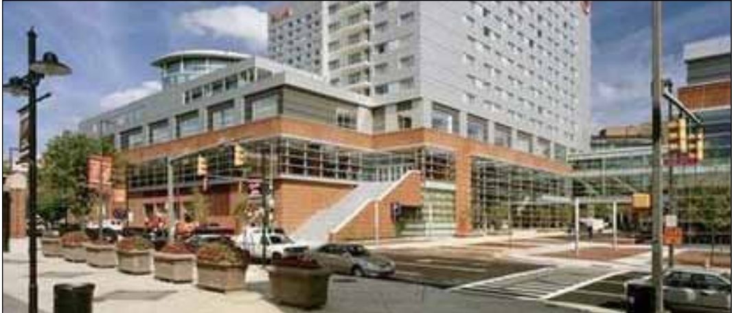
Hilton Convention Center Hotel - Baltimore, Maryland
