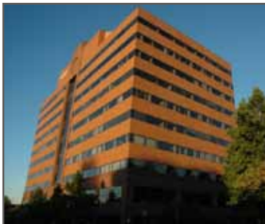
Bank of America Financial Center Vancouver, WA
