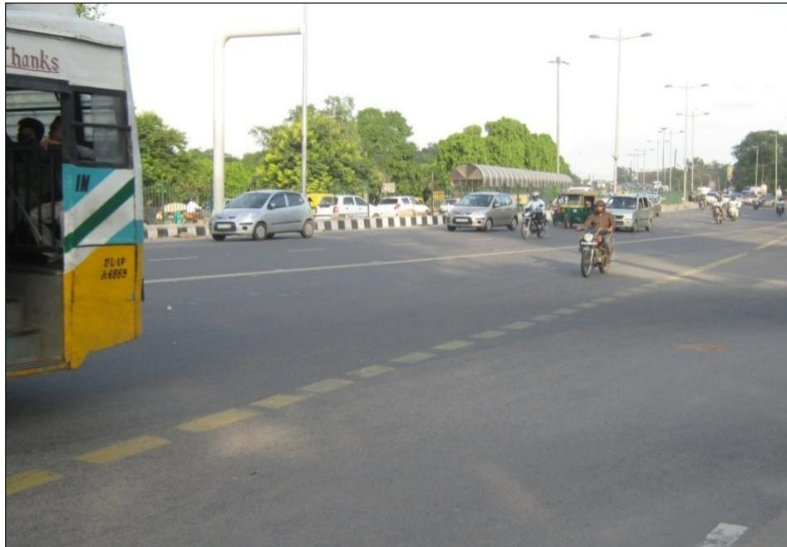
Figure 2.1 View of Kashmiri gate
