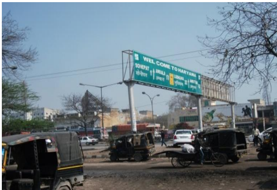
Figure 2.3 View near Kundli
