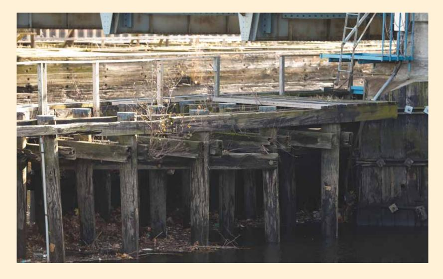
and rust in its steel elements, erosion around the underwater support piers, and corrosion to floorbeam sections. Mechanical problems with the swing bridge have been compounded by the fact that some replacement components are no longer available, which has led to the use of patches for repair work or alternate
