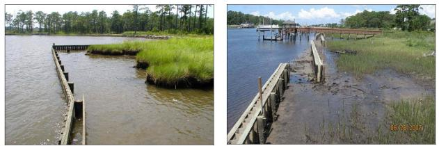
Figure 4. Examples of Sheetpile Sills Constructed from Timber (left) and Vinyl (right).
