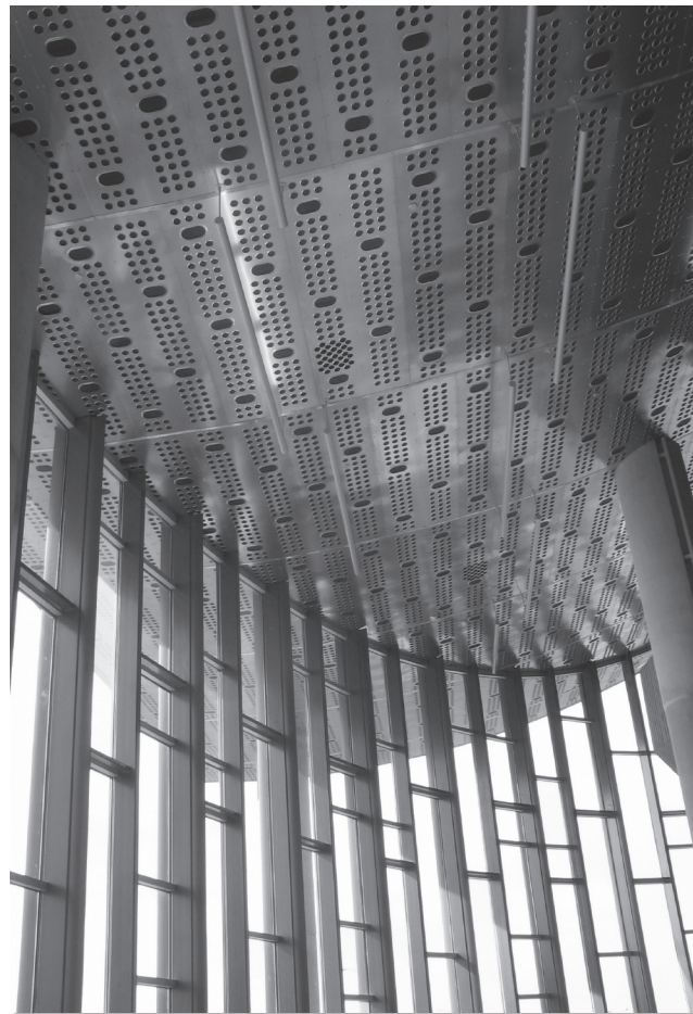
Cattle car siding finds reuse as ceiling tiles at the Amarillo Performing Arts Center in Texas. Photo ©Hands On! Inc.
