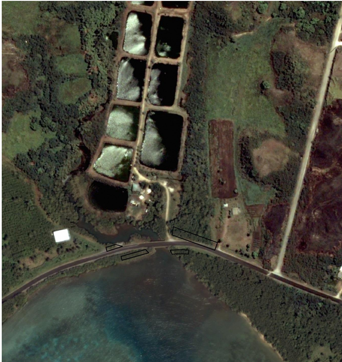
Figure 2. Ajayan Bridge Replacement Project Site
