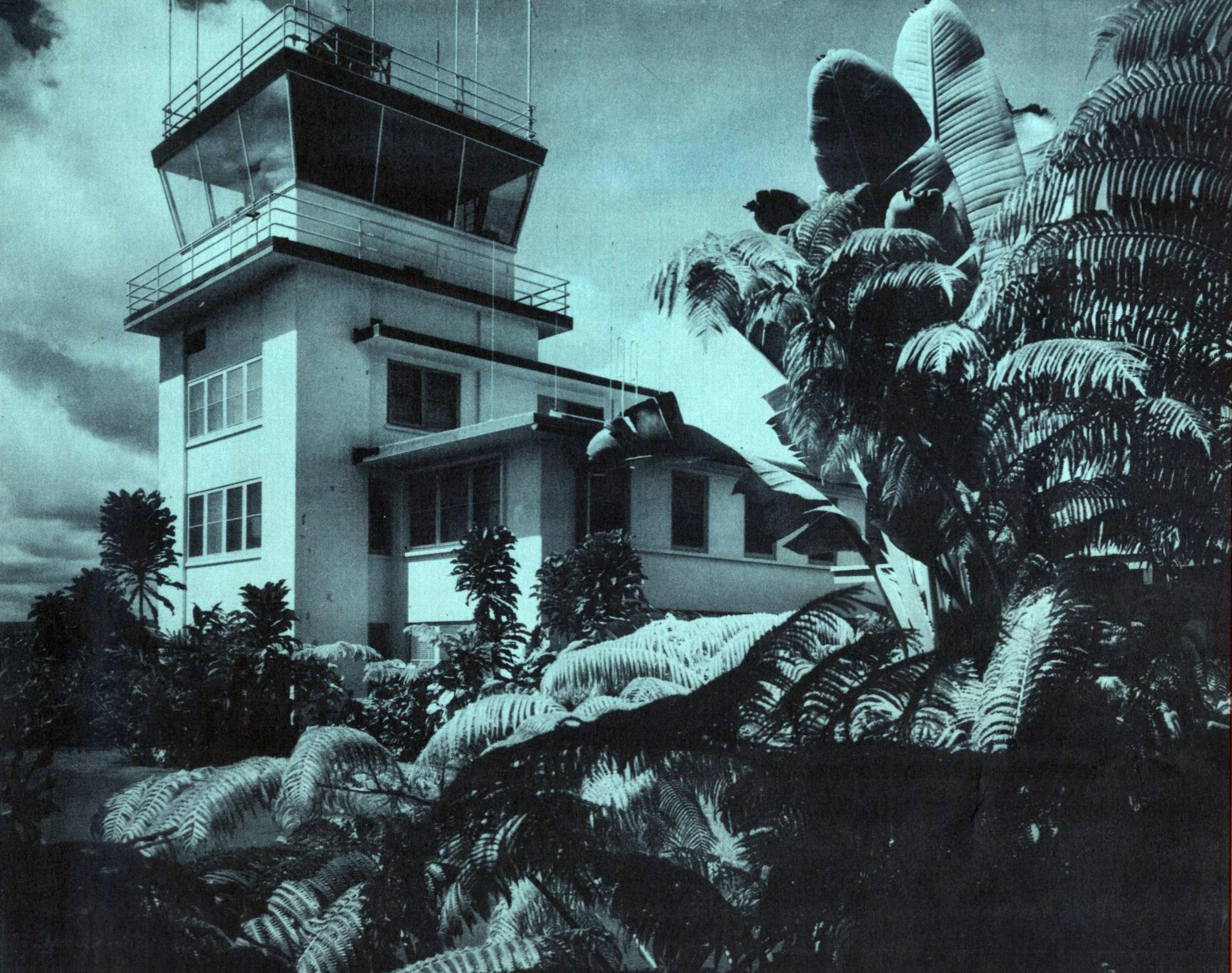
Hilo control tower with its setting of beautiful, lush tropical gardens.
